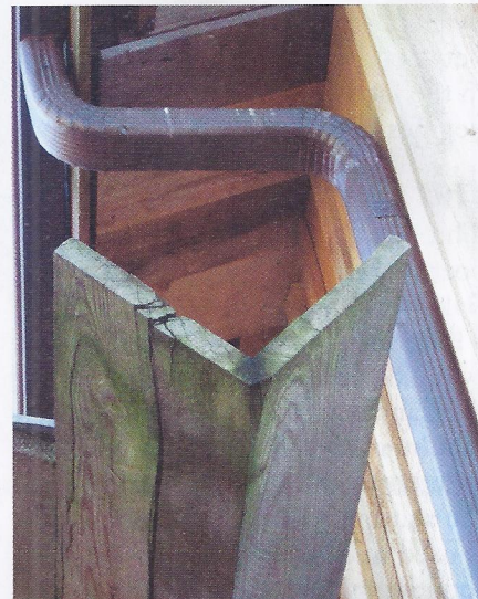
A joint-free wooden gutter made with a swingblade sawmill.
